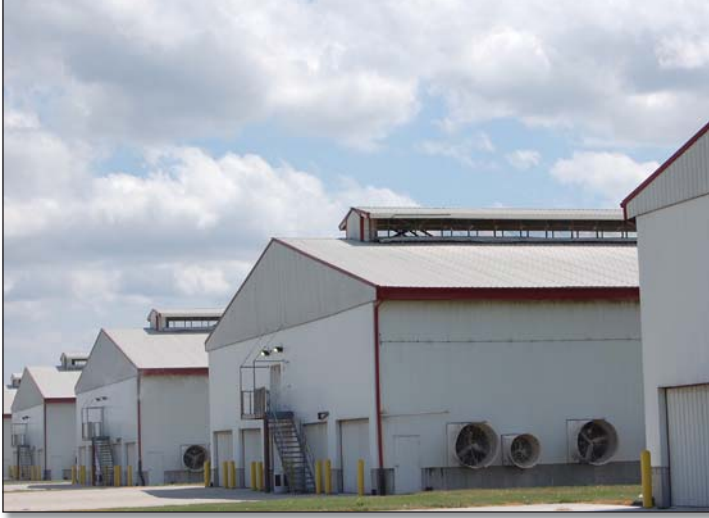
There are 12 identical high rise barns at the complex which house 280,000 layers each.
