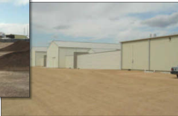
Newly erected aviary houses equipped with Salmest installations.
