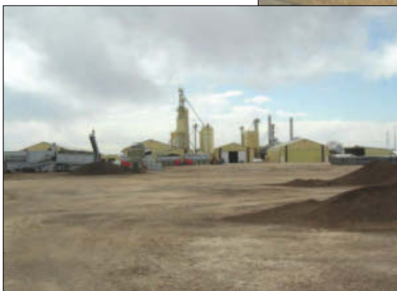
View of gas-fueled manure processing plant with rotary kiln.
