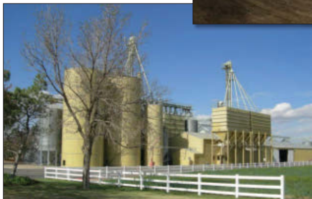
Dedicated feed mill for Morning Fresh complex with adequate ingredient storage and computerized control system.
