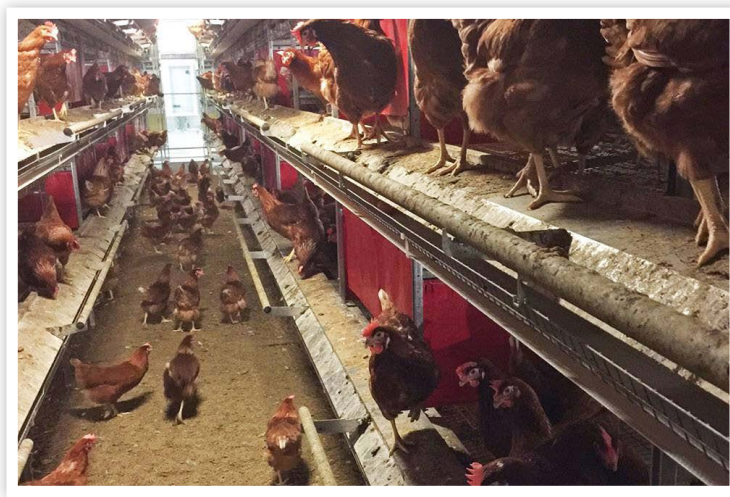
Allowing enough space in the aisleways for bird activity and worker movement through the system is an important consideration when placing aviaries in a house. | Courtesy Tecno Poultry
